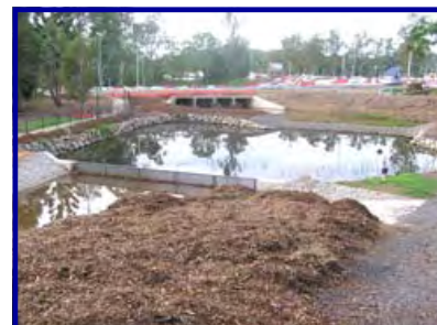
Stormwater Quality Improvement Devices at Ferny Grove
