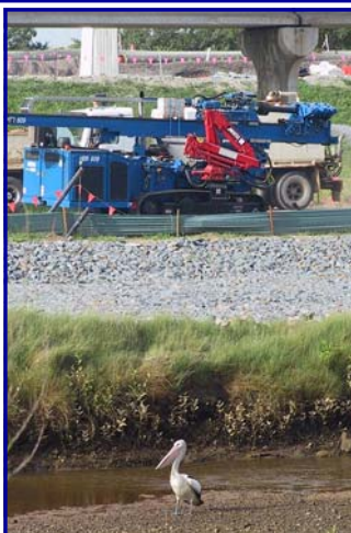
Lone pelican wanders through Toombul “flood mitigation” area. (R S-W)
